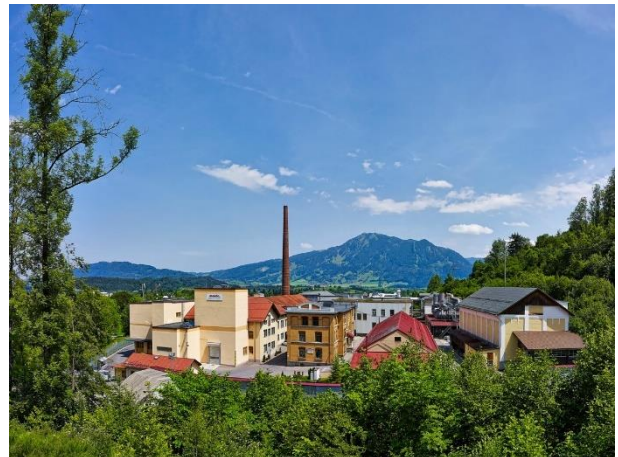
The monta company headquarters and production site, at the foot of the Alps, surrounded by unspoilt nature, on the outskirts of Immenstadt in the Allgäu region.
